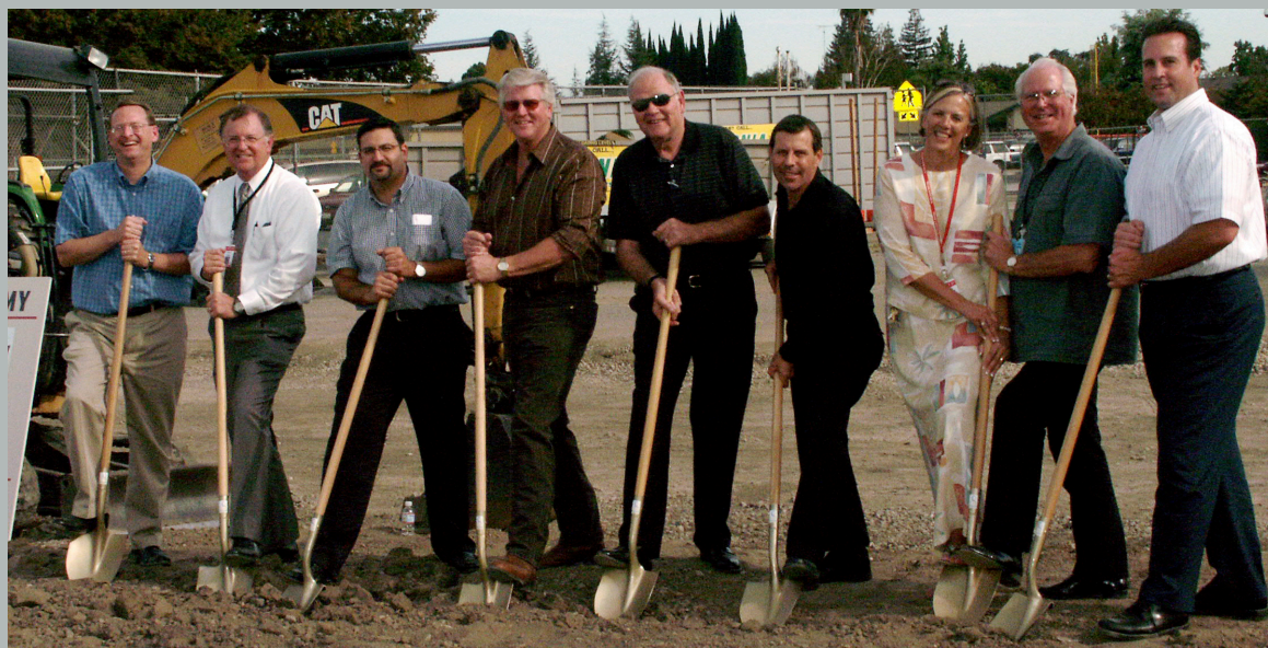
THE BOARD OF TRUSTEES AND SUPERINTENDENT LOWDER JOINED WITH TEACHERS JEFF WRIGHT AND DAVE DABACO, PRINCIPAL DEBBI HOLMERUD, STUDENTS, AND COMMUNITY PARTNERS TO CELEBRATE THE ENGINEERING AND CONSTRUCTION ACADEMY GROUNDBREAKING.
